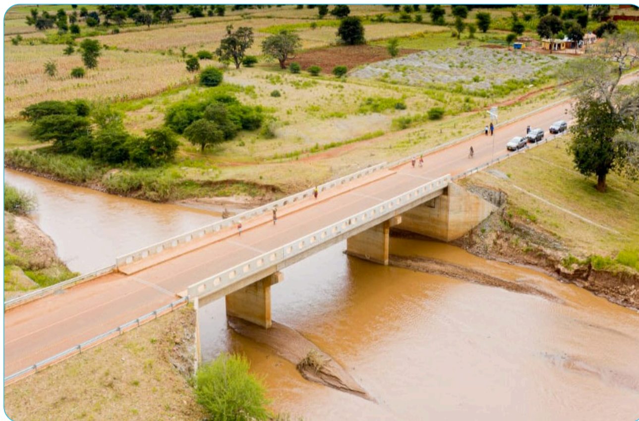
Momba Bridge across Momba River is one of new infrastructures in Songwe Region (Photo: Tanroads)
